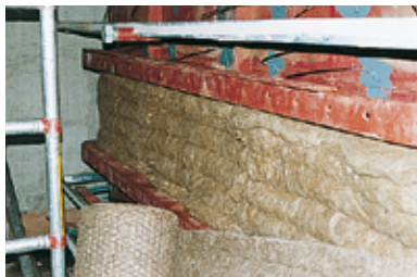
5. Place the pre-insulation layer on top of the mineral wool.
