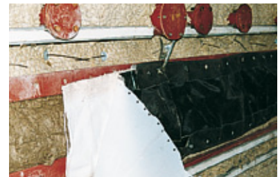
6. Assembly of the multilayer expansion joint.
