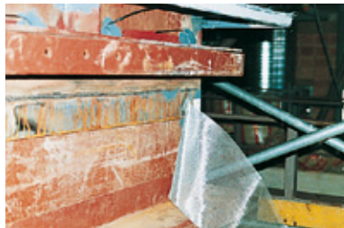
2. V4A alloy mesh to be folded on each side ...
