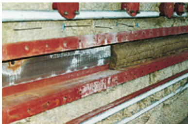
4. Mineral wool is installed.
